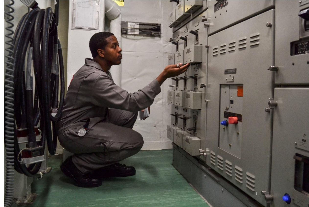
171205-N-IR859-229 ATLANTIC OCEAN (Dec. 5, 2017) Senior Chief Electrician's Mate Franklyn Munroe, an inspector from the Board of Inspection and Survey (INSURV), inspects a load center aboard the guided-missile destroyer USS Cole (DDG 67). Cole is underway conducting INSURV, which is a periodic inspection to ensure the ship meets Navy standards. (U.S. Navy photo by Chief Mass Communication Specialist Jen Blake/Released)
