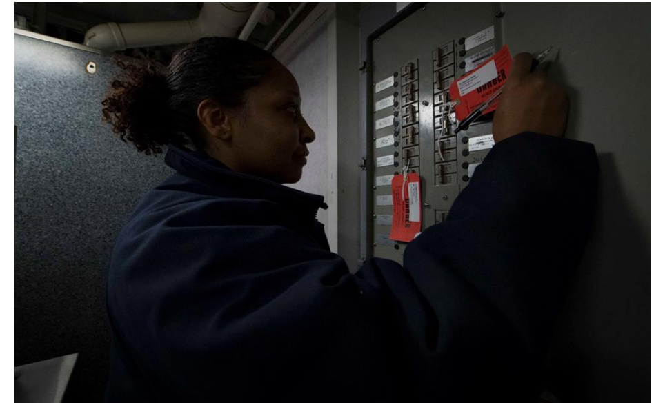
170425-N-HV059-034 NORTH SEA (April 25, 2017) Machinist's Mate 3rd Class Zaeeda Walters verifies that a power control panel has been properly tagged out aboard the guided-missile cruiser USS Leyte Gulf (CG 55). The ship is conducting naval operations in the U.S. 6th Fleet area of operations in support of U.S. national security interests in Europe. (U.S. Navy photo by Mass Communication Specialist 2nd Class Sonja Wickard/Released)
